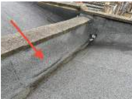
Photo 8 - Air pockets and untidy felt
