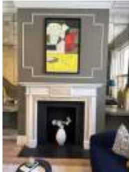
Photo 123 - Suspected false fireplace
