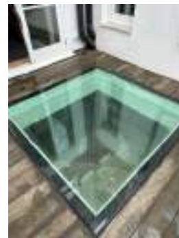
Photo 13 - Rooflight leaking
