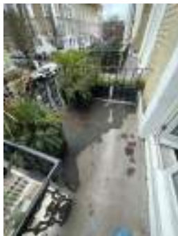
Photo 16 - Front portico roof
