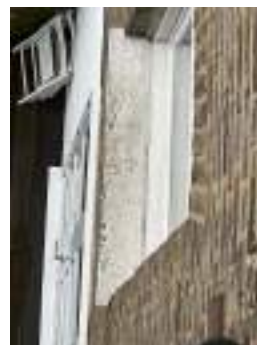
Photo 45 - Weathered and crack to paint with poor seals to window sill Photo 46 - Weathered and crack to paint with poor seals to window sill
