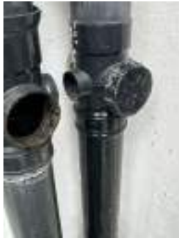
Photo 154 - Leaking joint
