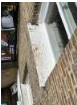
Photo 45 - Weathered and crack to paint with poor seals to window sill Photo 46 - Weathered and crack to paint with poor seals to window sill
