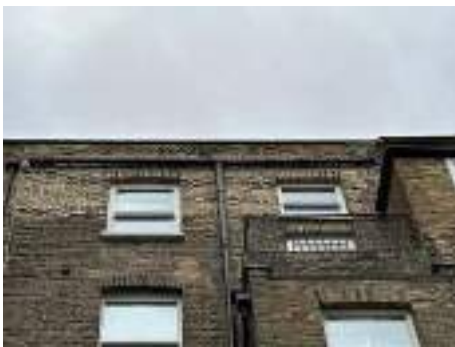
Photo 57 - Upper section of the walls rebuilt
