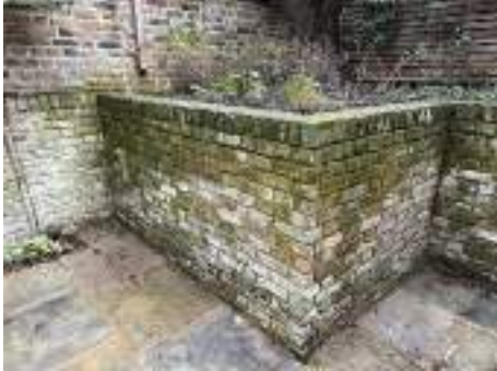
Photo 85 - Water staining
