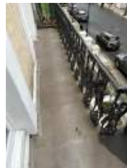
Photo 15 - Front balcony roof
